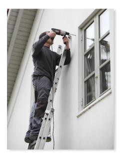
8. When the ladder hangs in the top hole, the ladder is placed in exact vertical and the drill holes are marked up.
