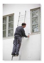
11. The ladder is installed again and the mounting screws are tightened. It is recommended to install the top bracket first and then continue down.
